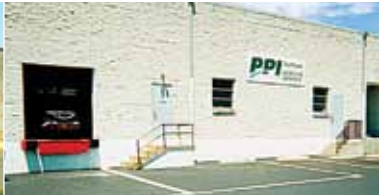
Northeast Service Center Lewisberry, PA
